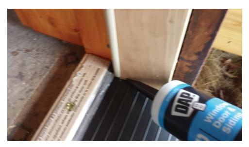
Apply a bead along the front edge of the seal and the cover. (On sills with no seal, adjust the rail properly and add the bead to the intersection between the rail and the cover).
