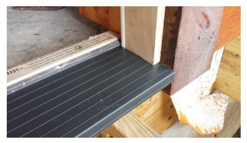
TIP: Press into place. Make sure to press along every square inch of the cover to properly set it in place. Some squeeze-out of the adhesive may occur. Clean it up immediately using a towel or rags. It is recommended that you temporarily tape the sill cover in place and over the sill rail. This will keep it from sliding forward until cured. Allow 24 hours before allowing any direct traffic across the sill (step over, but not on!)
