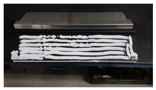
TIP: Apply a liberal and continuous bead between each tread on the underside of the cover. Also remember to add a bead on the front edge.
